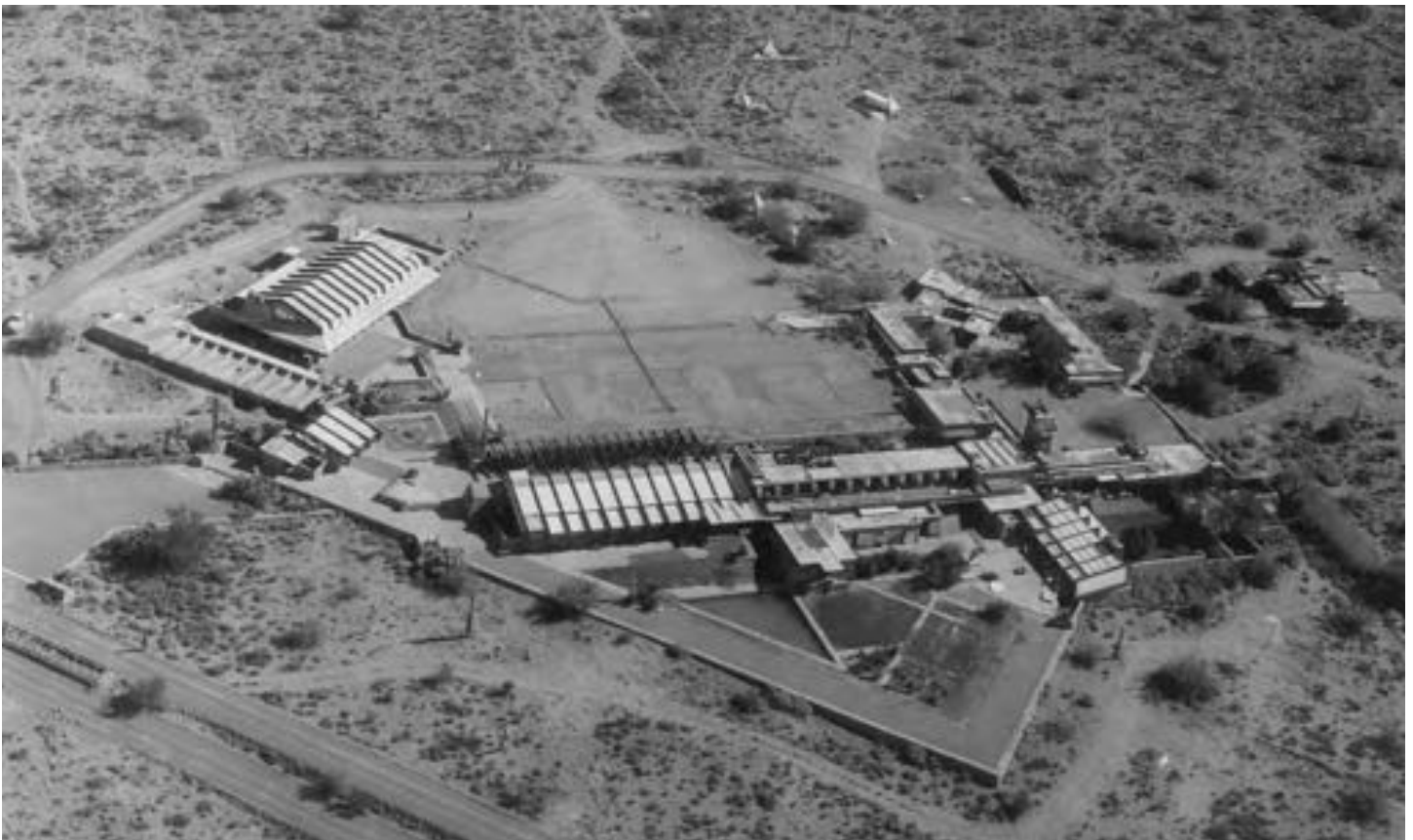
Figure 10-1 - Aerial view of Taliesin West, 1959 (Pedro Guerrero).
