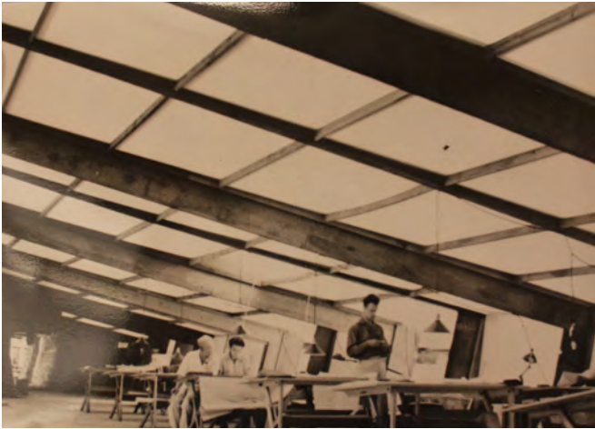
Figure 6-7 - Canvas roof overhead in Drafting Studio, ca. 1939 (The Frank Lloyd Wright Foundation Archives, The Museum of Modern Art | Avery Architectural & Fine Arts Library, Columbia University, New York).
