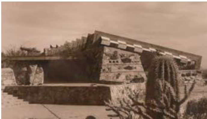
Figure 8-1 - West end of Drafting Studio, ca. 1958 (The Frank Lloyd Wright Foundation Archives, The Museum of Modern Art | Avery Architectural & Fine Arts Library, Columbia University, New York).
