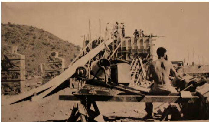
Figure 6-5 - Construction of Kitchen and Drafting Studio, ca 1938 (The Frank Lloyd Wright Foundation Archives, The Museum of Modern Art | Avery Architectural & Fine Arts Library, Columbia University, New York).
